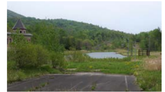
Former National Highway 230: The 2000 eruption lifted the ground surface, disrupting traffic and ultimately turning the area into a swamp.
